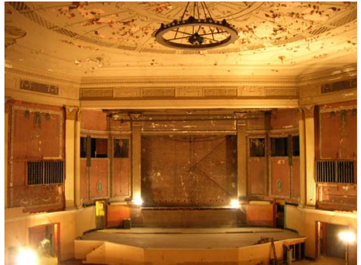
Interior of Capitol Theatre under renovation
